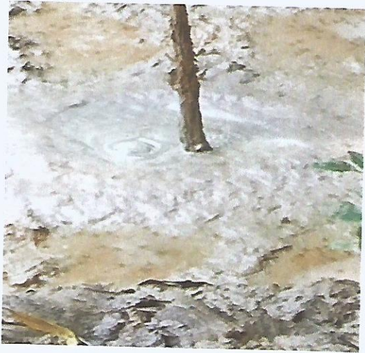
Fig 1. Showing the incident point before excavation.
